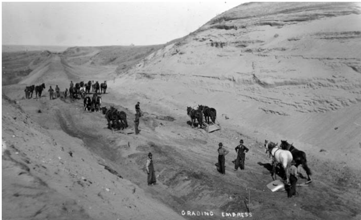
This photo is described by Edgar Potts: "The making of a railroad, a very dusty job on a windy day." The image looks down on a team of horse and men plowing the dirt for the railroad. [ca.1912 - 1913] From the Esplanade Archives. Accession Number: 0817.0008
